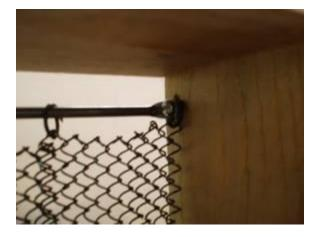
Thread the curtain onto the rod. Then, lining up the last curtain ring (the ring farthest from the center) with the hole in the end of the rod, attach each into the side of your fireplace opening. This will ensure that the screen curtain does not slide into the middle.
