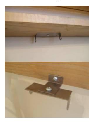
Attach the center bracket (or the combined brackets, for arched fireplaces) to the lintel using either a lag bolt for your masonry fireplace or a metal screw for your metal firebox.
